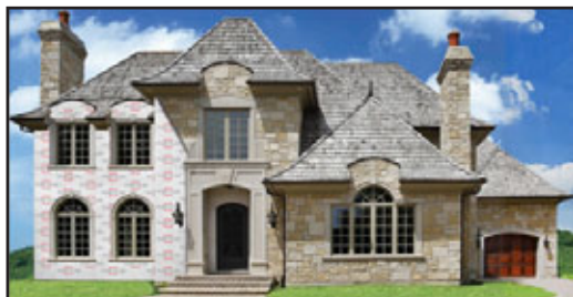
Below - Picture 4: House built with Cemex's Fortium ICF.
